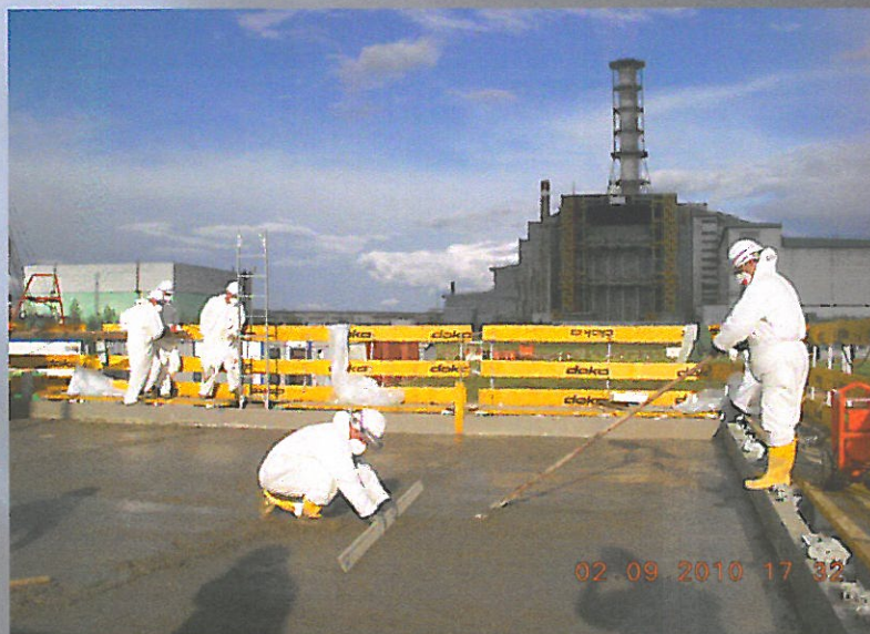
Industrial Zone Foundation - Concreting
